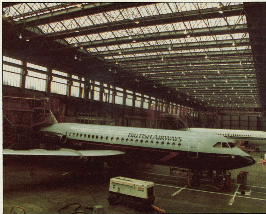
A view of British Airways' refurbished hangar at Heathrow.
