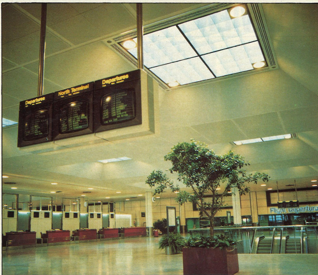
The departure lounge uses a combination of linear and compact fluorescent fittings.
